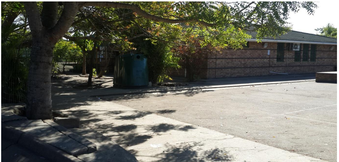
Figure 3: Picture of school used in the study – Original building
