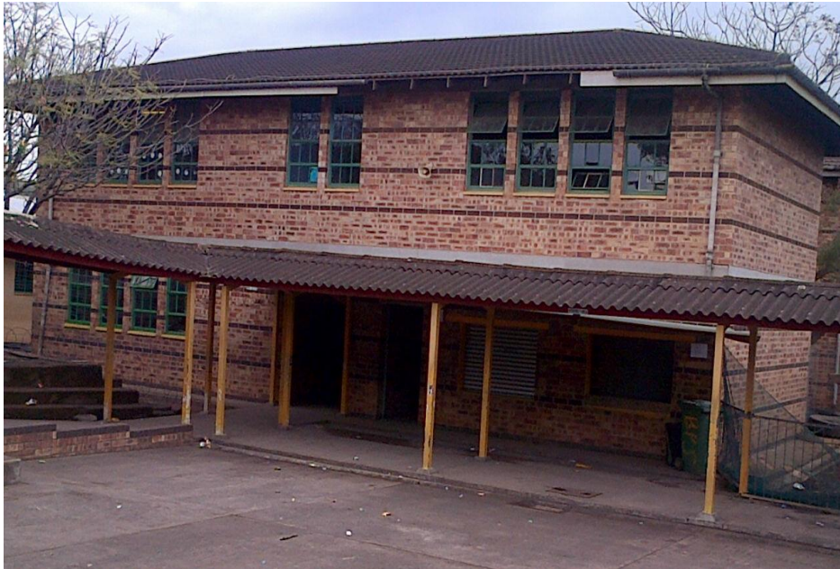
Figure 2 : Picture of school used in the study – original classrooms
