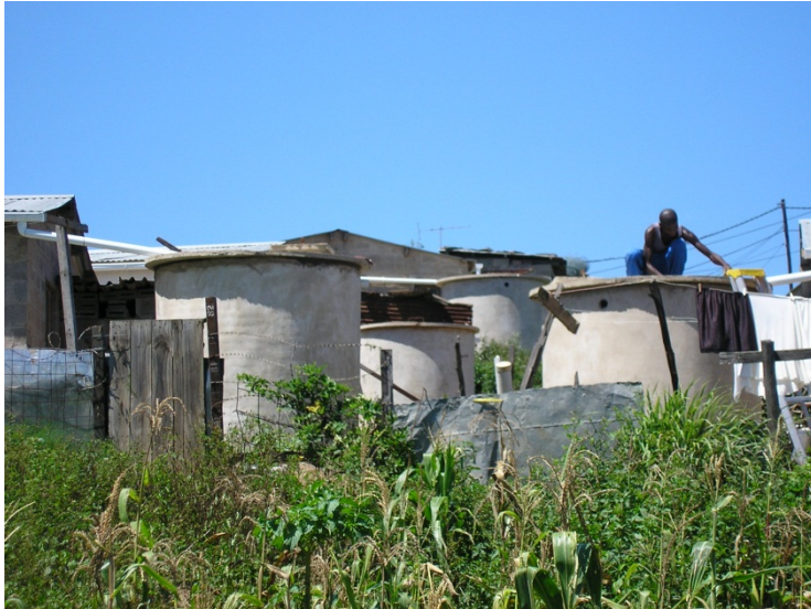
Figure 6.2: Household rain water harvesting for irrigation
