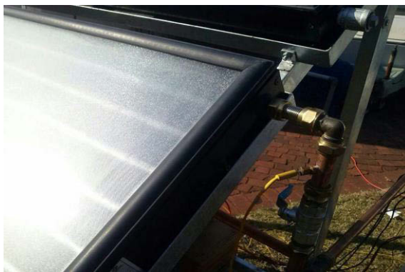
(c) Thermocouple on vertical pipe
