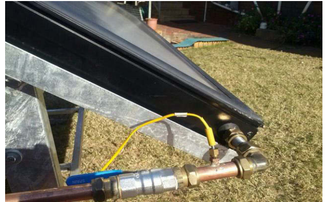
(b) Thermocouple on horizontal pipe
