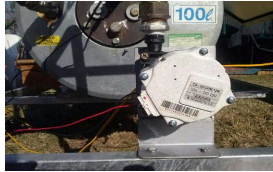
(b) Pump installation
