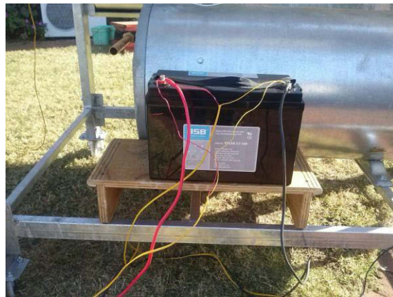
(b) Battery Installation
