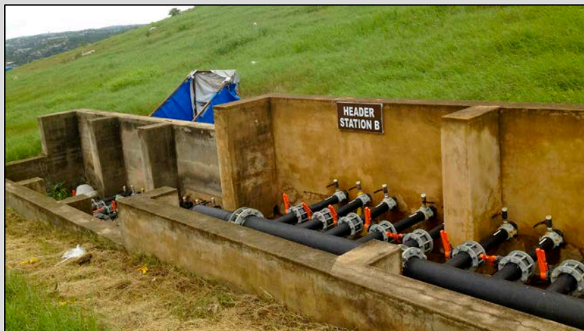
Figure 2 - 6: Header Station for Pipe Control
