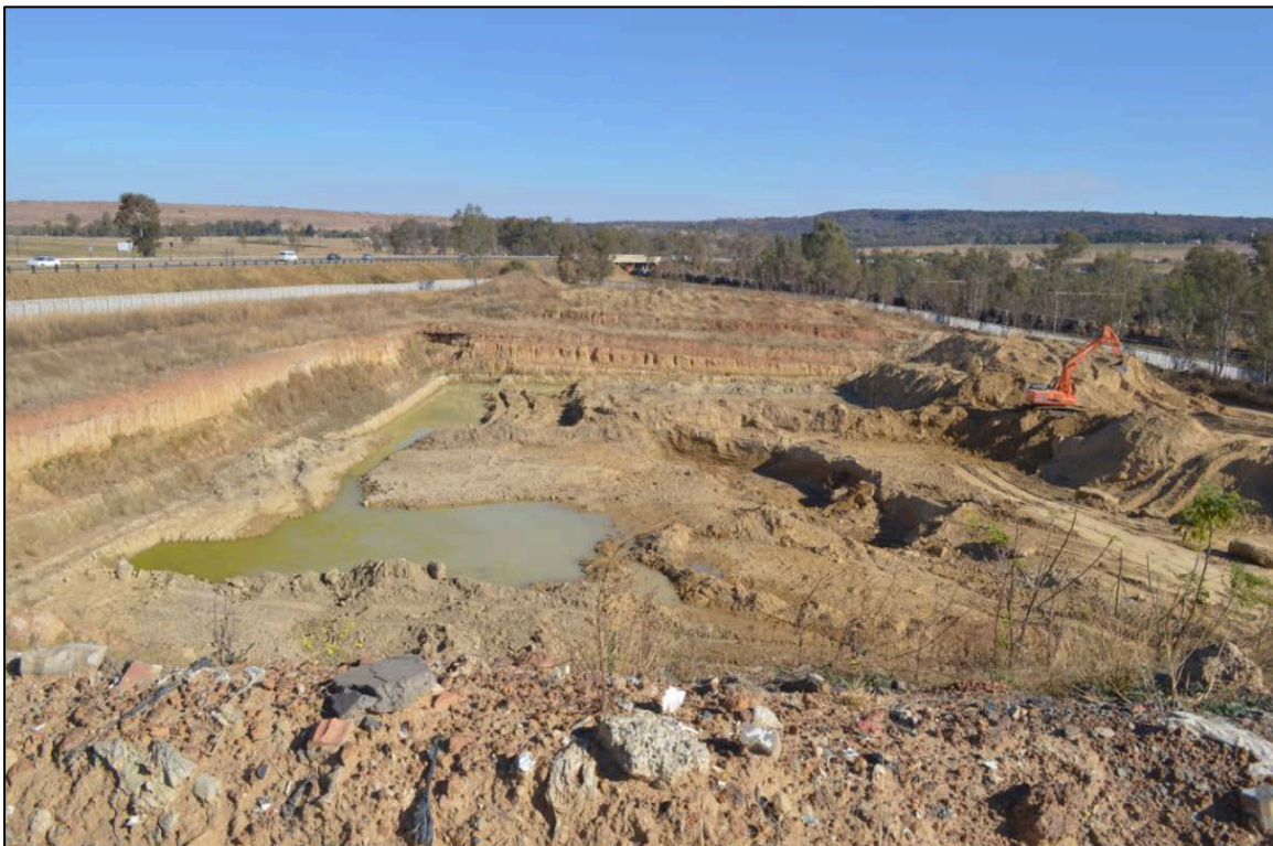
Figure 4 - 8: NLM Landfill New Cell
