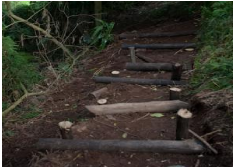
(a) Contouring and reinforcing using logs on trails
