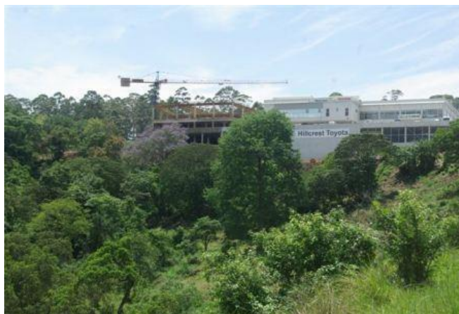
Figure 5.8: Toyota Dealership development (Source: Field photographs)
