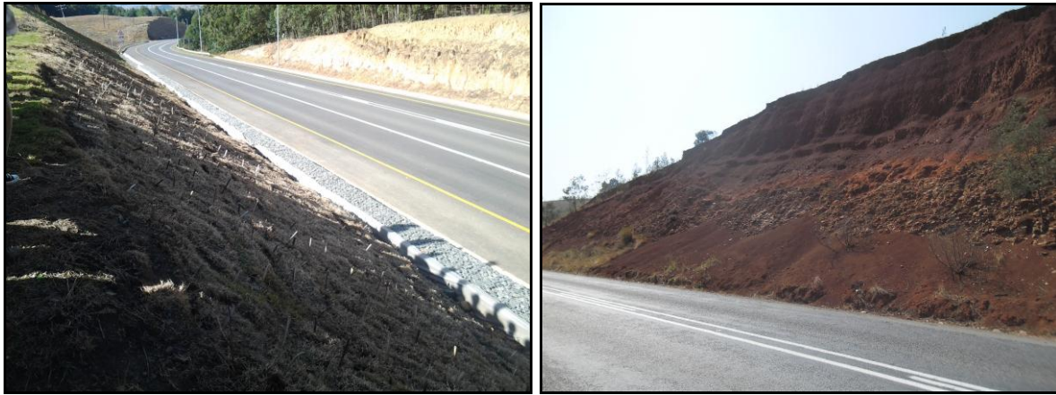
Figure 2. 2: (a) Successful application of vegetation cover to control erosion on a roadside slope and (b) signs of erosion on a roadside slope due to the absence of vegetation cover.
