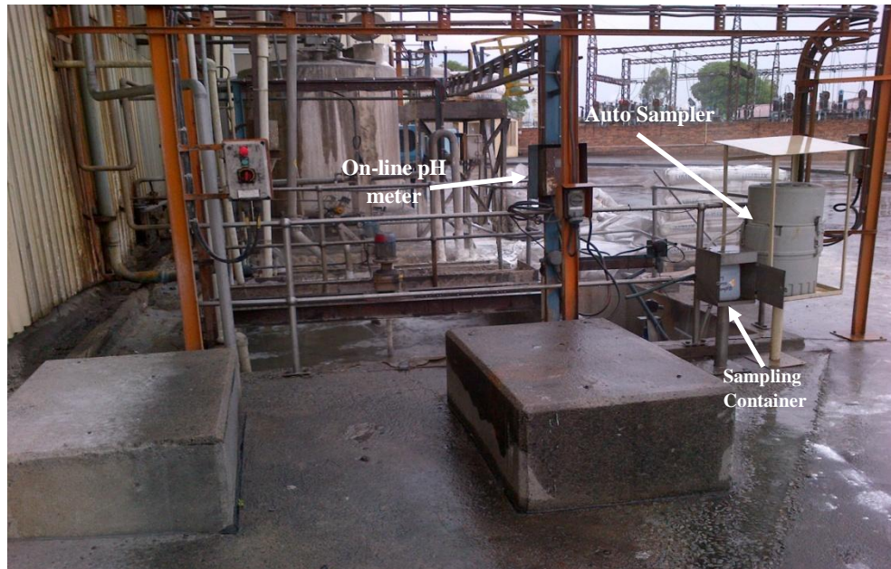
FIGURE 3-5a: E7 Effluent monitoring system (E&H ISCO 3700 Auto sampler)
