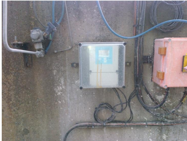
FIGURE 3-7: Anaerobic digester feed on-line pH monitoring (E&H Liquisys M CPM transmitter)
