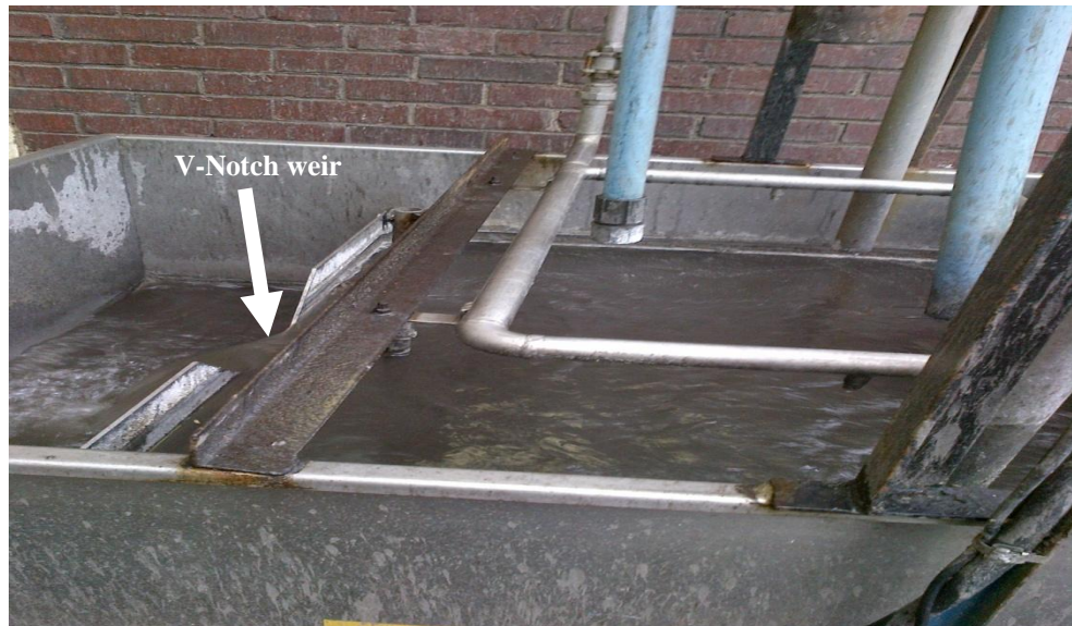
FIGURE 3-4a: E4 90° V Notch weir flowmeter
