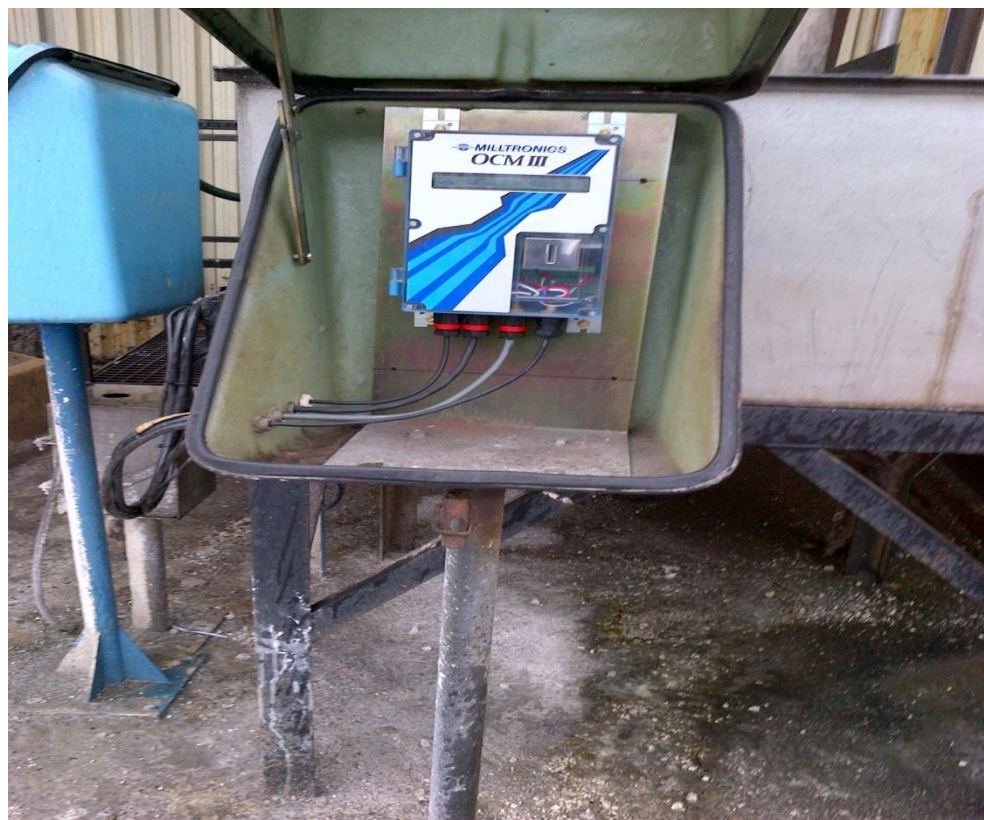
FIGURE 3-4b: E4 flow transmitter
