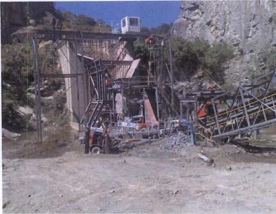
e) Primary crusher, where the sorting out of rock occurs.
