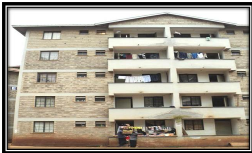
Figure 5: Building in Lang'ata decanting site
