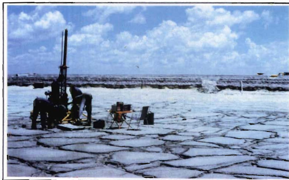
CPT RIG AT PLATINUM TAILINGS DAM - BAFOKENG.
