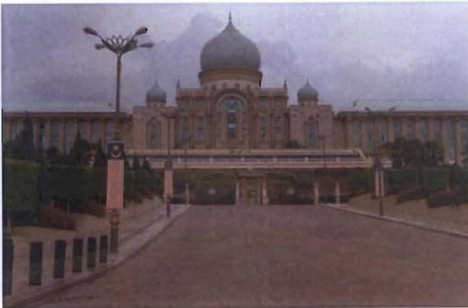
Illustration 14 Putrajaya Building in Malaysia a literal symbol of the country's culture with the use of domed towers, and the verticality of the window panes with columns emerge thereof.
