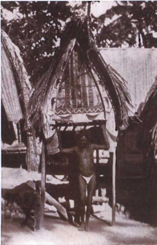
Illustration 15. Papua New Guinea. A pointed roof hut to allow water to run-off, with the suspended base to allow rain water to run below without destroying the structure.
