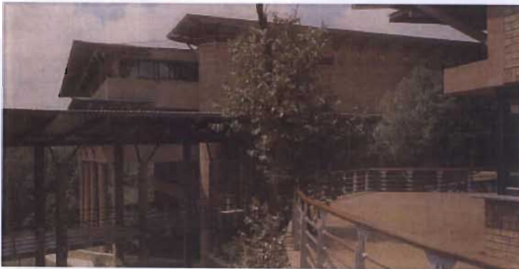
Illustration 58. Linking bridges and timber deck: Simplicity of structure and practical response to local climate Source: Planning, 174, March/ April, 2001, p.49
