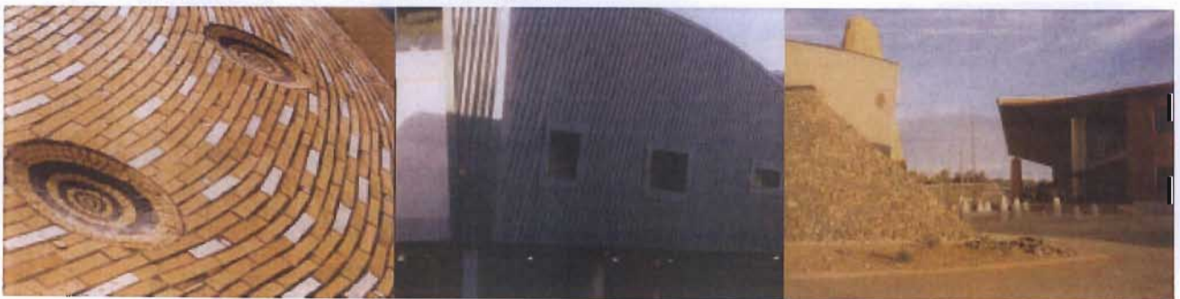
Illustration 53. Corrugated Iron Sheetting, common brick and reinforced concrete are the primary materials applied during construction
