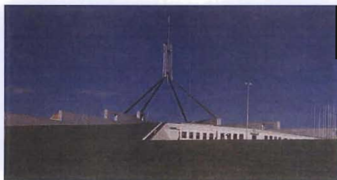
Illustration 32. View from the public green space above the structure Source: Architecture Australia, 1988, p.83
