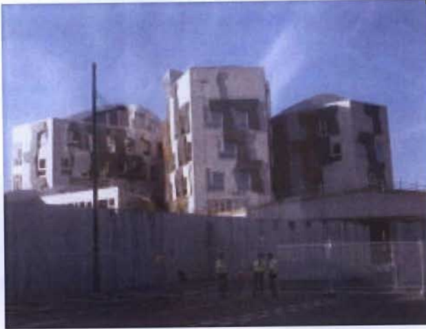
Illustration 47 Parliament Facade with trigger panels to windows Source: www.en.wikipedia.org/wiki/Scottish_Parliament_Building April 2008
