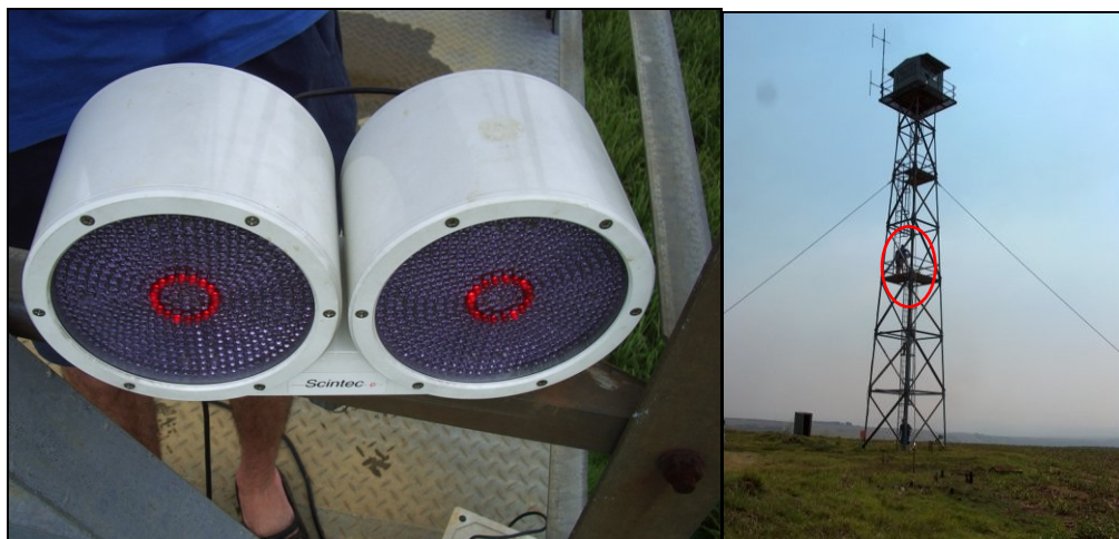
Figure C1: BLS 900 transmitter (left) and fire tower on which it was mounted (right)
