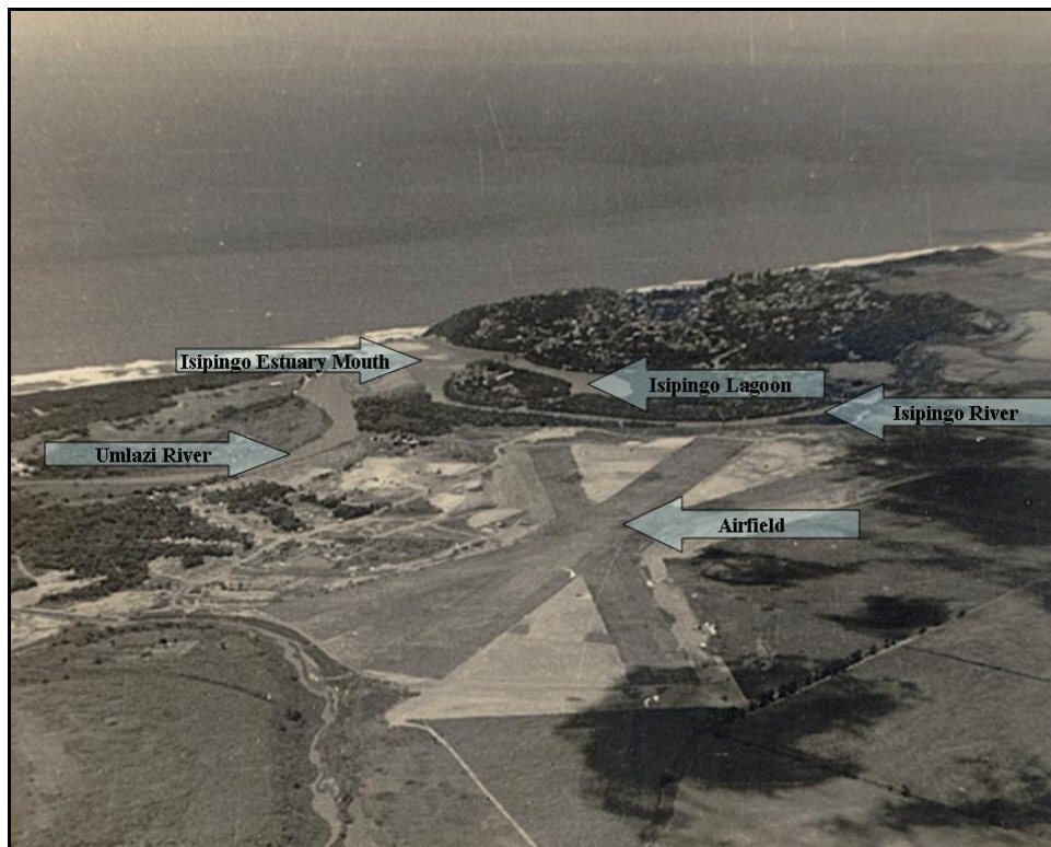
Figure 1.11: Isipingo Estuary and Umlazi River in 1942 (after eThekweni Municipality, 2010)
