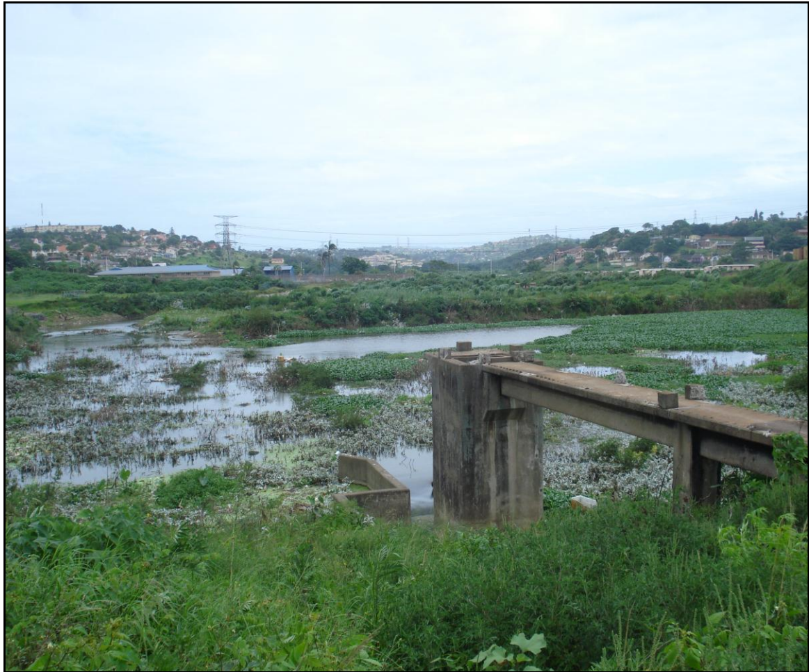
Figure 1.12(b): The Diversion Works System (2010) showing the large concrete structure which houses the sluice gates that allows pooled water to flow into the PCS. Water hyacinth is present in the background (Taken on 16 November 2010)
