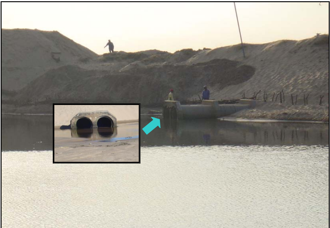
Figure 1.6(b): Photograph showing tidal inlet pipes on the estuarine side. Dune barrier separating the estuary from the marine environment
