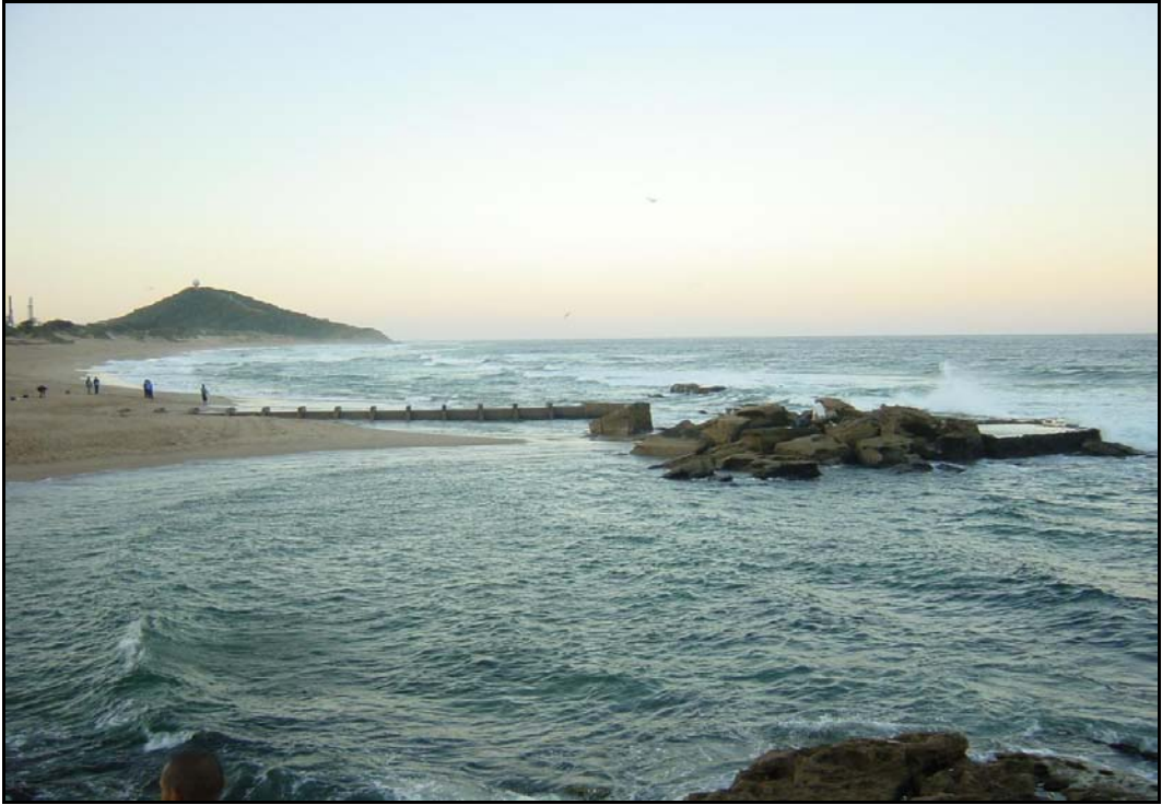
Figure 1.6(a): Photograph depicting the twin concrete pipes maintaining connectivity between the estuary and the sea
