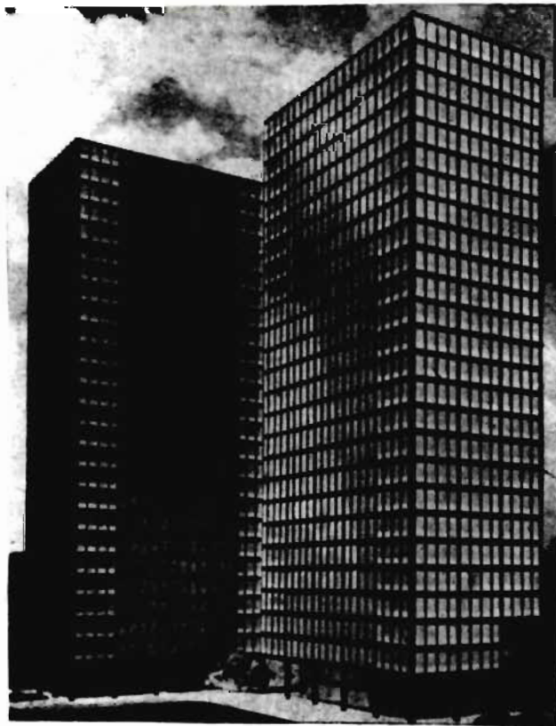
Fig.21. Lake Shore Drive Apartments, Chicago.
