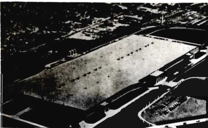
Fig. 38. Factory without windows.
