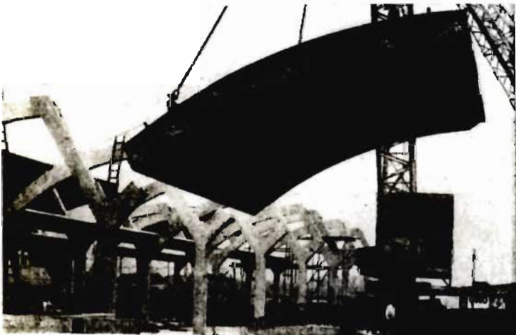
Fig. 36. Prefabricated structure and roof panels.
