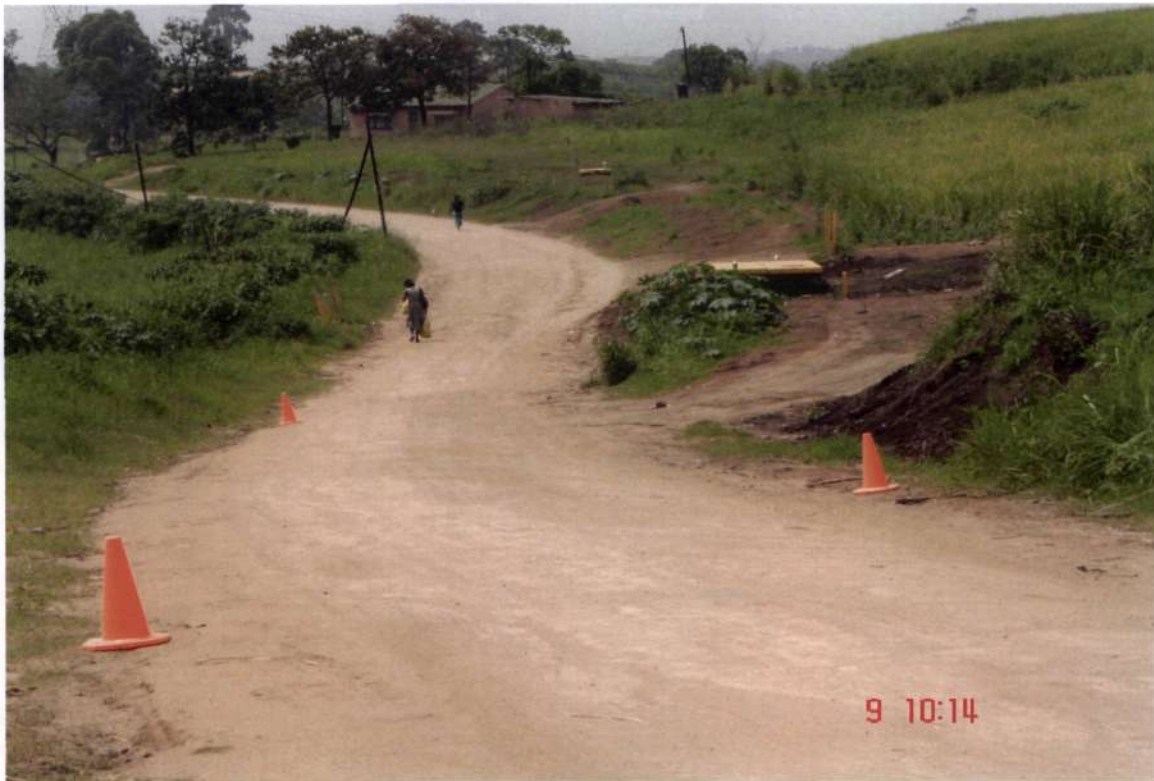
Image 4.2: Maintained Rural Road in Umbumbulu (D991)
